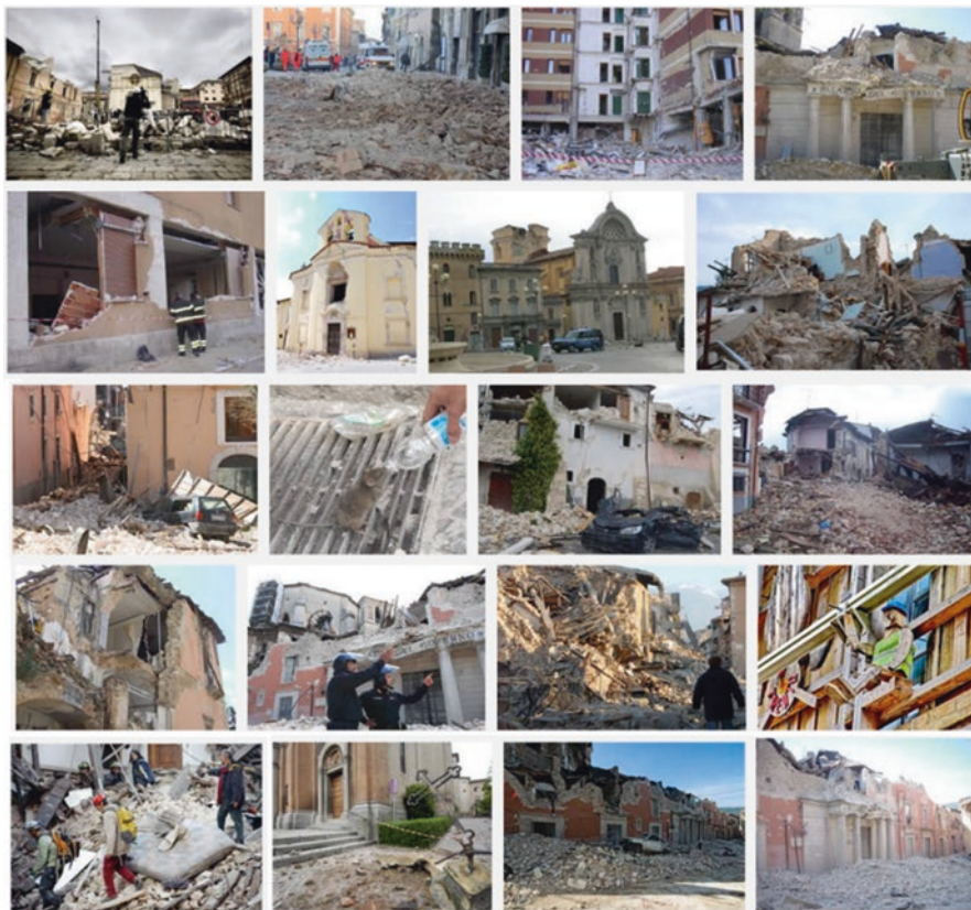
Fig. 3 Several scenes of L'Aquila historic centre, severely damaged during the earthquake occurred in 2009
